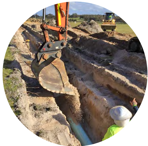
Our crew working on the Denmark pipeline
