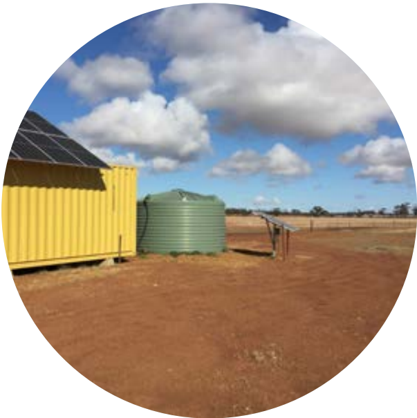
On-farm desalination plant in Burracoppin
