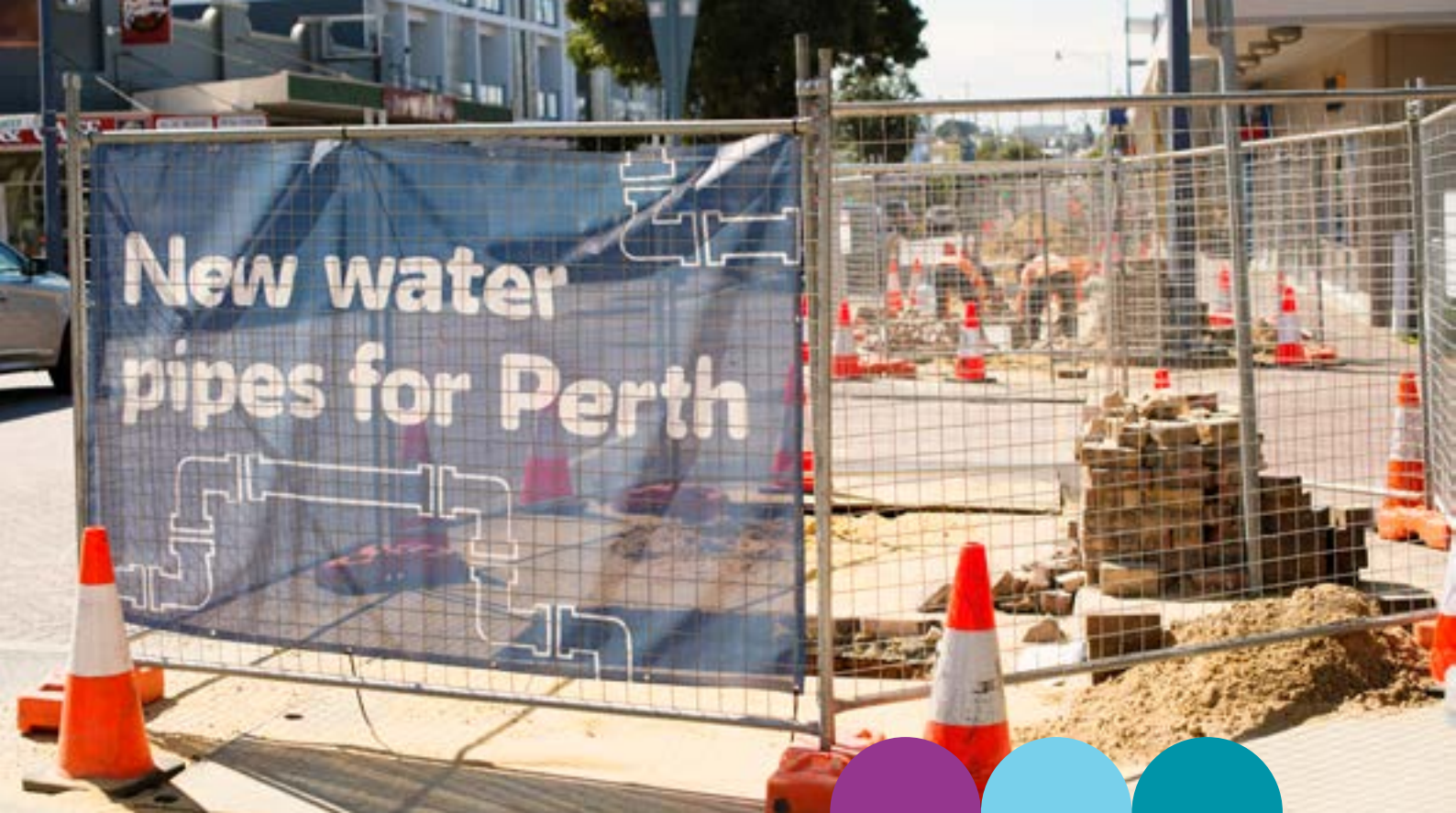
Pipes for Perth renewal Program.
