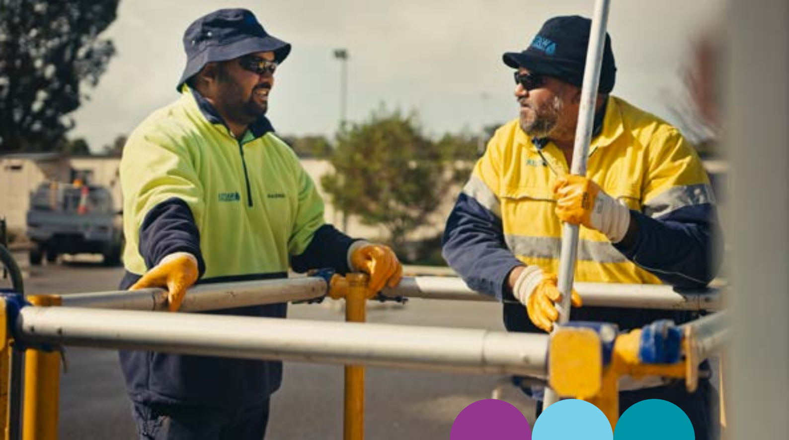
Completing upgrades in the South West.
