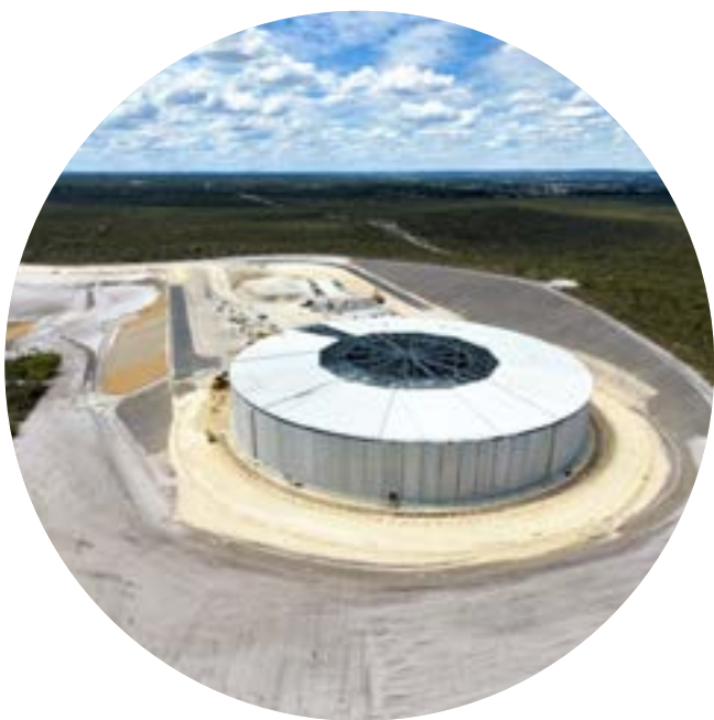
Ellenbrook Tank, our largest ever water storage tank.
