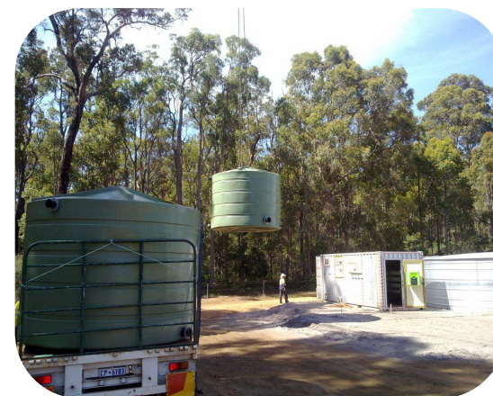
Preparing mobile UF plant
