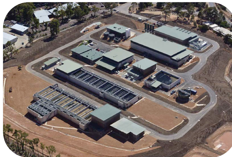
Mundaring Water Treatment Plant
