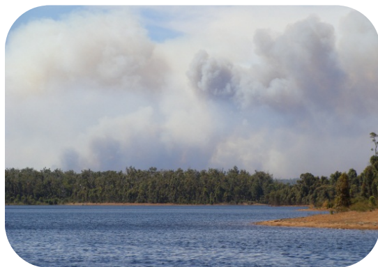
Harris Dam, South West Region
