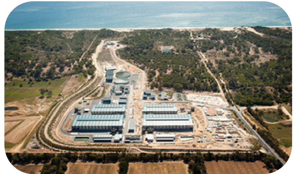
Southern Seawater Desalination plant, near Binningup
