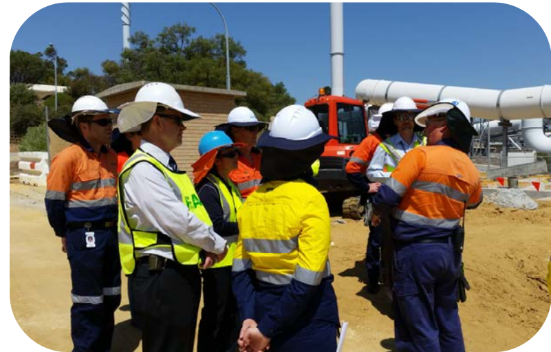
Department of Health and Water Corporation at AWRP construction site
