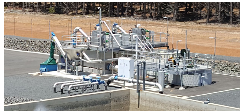
Figure 18: New inlet works and grit removal system
