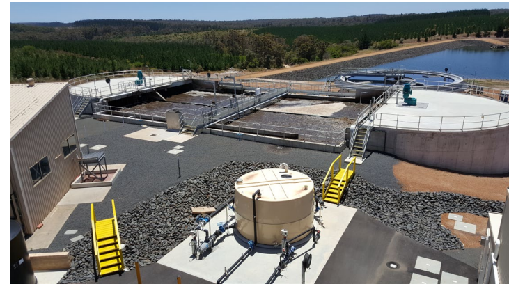
Figure 17: New Oxidation Ditch and Clarifier
