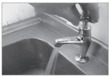
Fill sinks with clean water and empty to flush through unit. This keeps freshwater in tank. Always ensure water level is reaching wheels.
