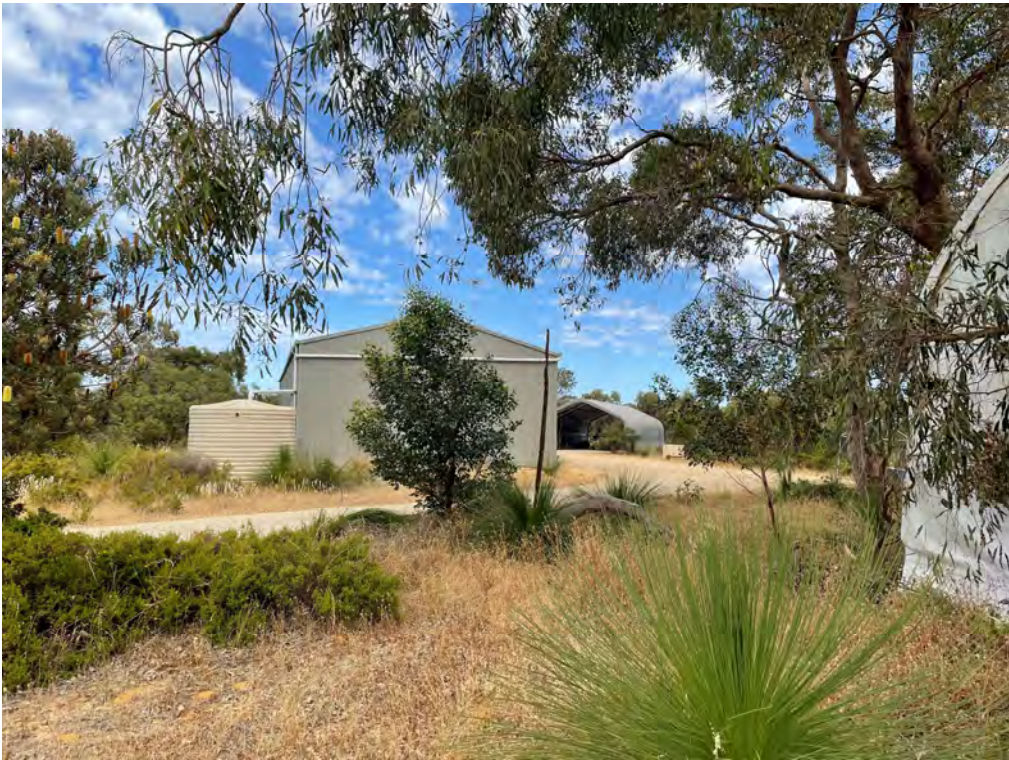
Figure 1. Shed with water tank and shade structure for vehicles behind.
