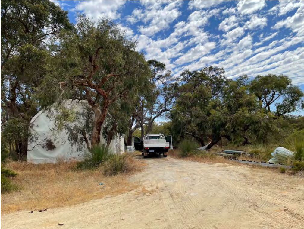
Figure 2. Shade structure over two shipping containers.
